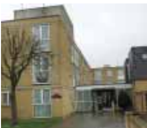
Owen House Shore Close Bedfont TW14 9QE
