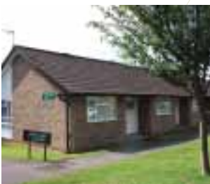
Rectory House Fernside Avenue Hanworth TW13 7QE
